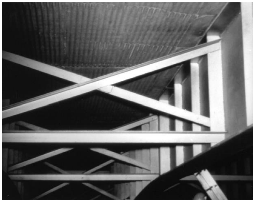
Figure 14 X-Bracing and Girders
